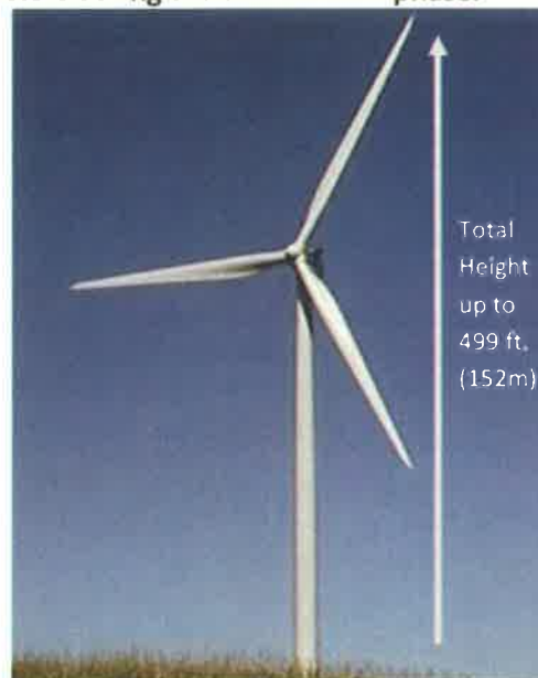
Figure 3: Wind turbine schematic with typical dimensions.
